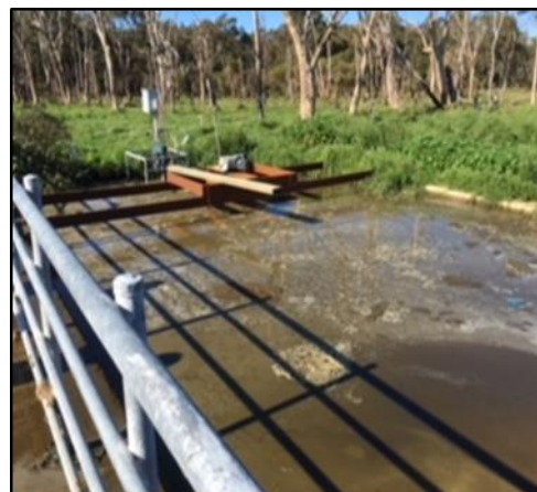
Typical Effluent Pond and Pump
