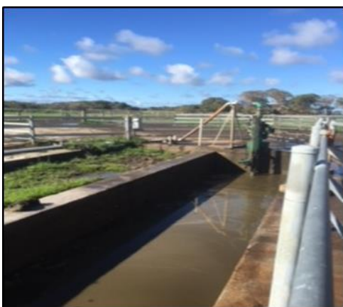
Similar Typical Effluent Pond and Pump
