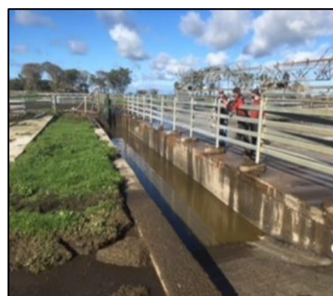
Effluent Pond with Choked Weeping Wall
